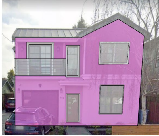
908 Cedar, Berkeley Openings are approximately 30%
